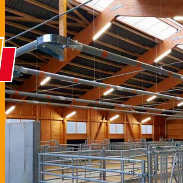
Distribution circuit with deflection corners
